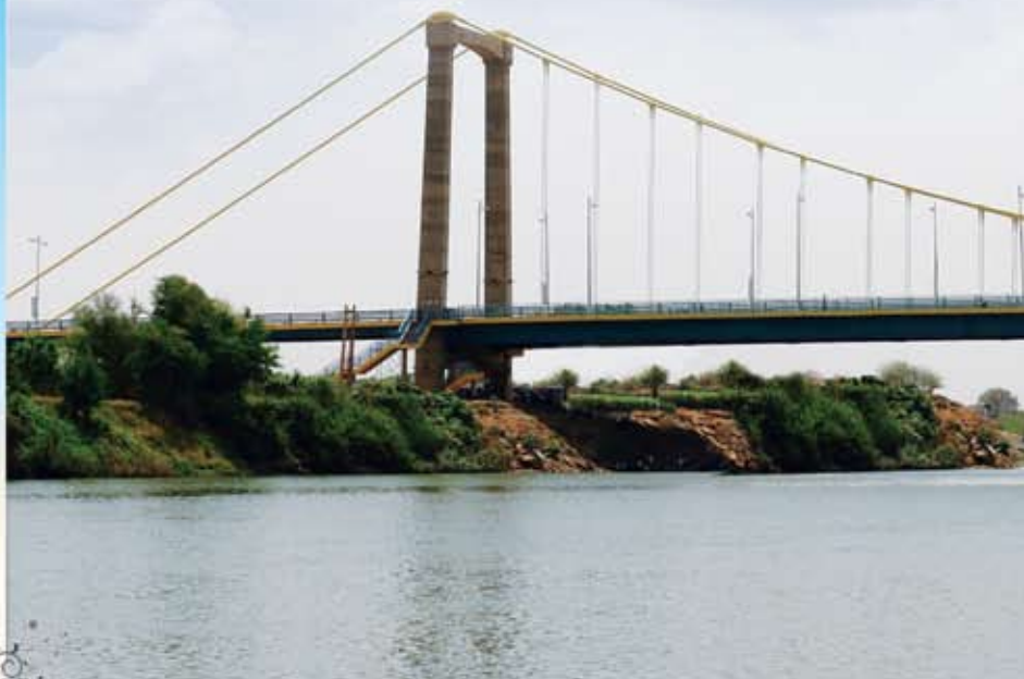
Tuti Suspended Bridge...a gateway for investment in a productive island
